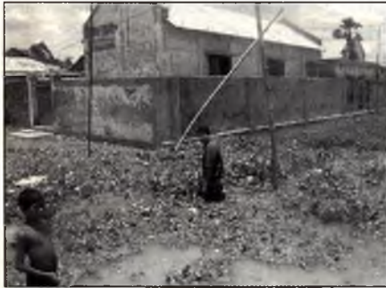
Nathan Biswas (right), national NCM coordinator, wades knee-deep in water as he evaluates flood damage at Nayanagar Church of the Nazarene in Bangladesh.
