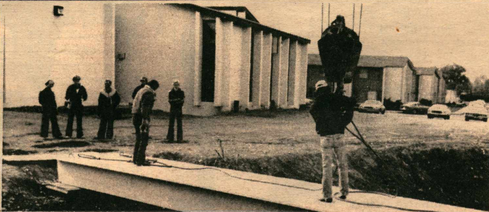
Maintenance department puts the finishing touches on the bridge over the infamous drain.
