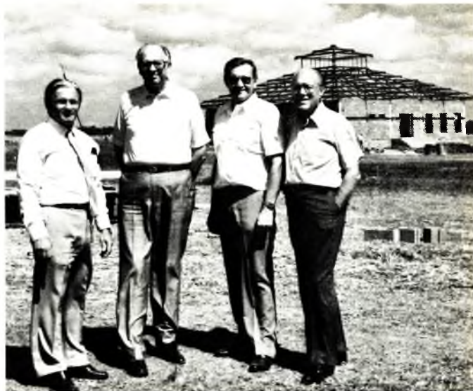
Nazarene administrators are photographed in front of the chapel that is being constructed at the proposed Africa Nazarene University in Nairobi, Kenya. Shown (l. to r.) are Harmon Schmelzenbach, East Africa field director; Jerald D. Johnson, general superintendent; Richard Zanner, Africa regional director; and Mark R. Moore, rector of the new school.
