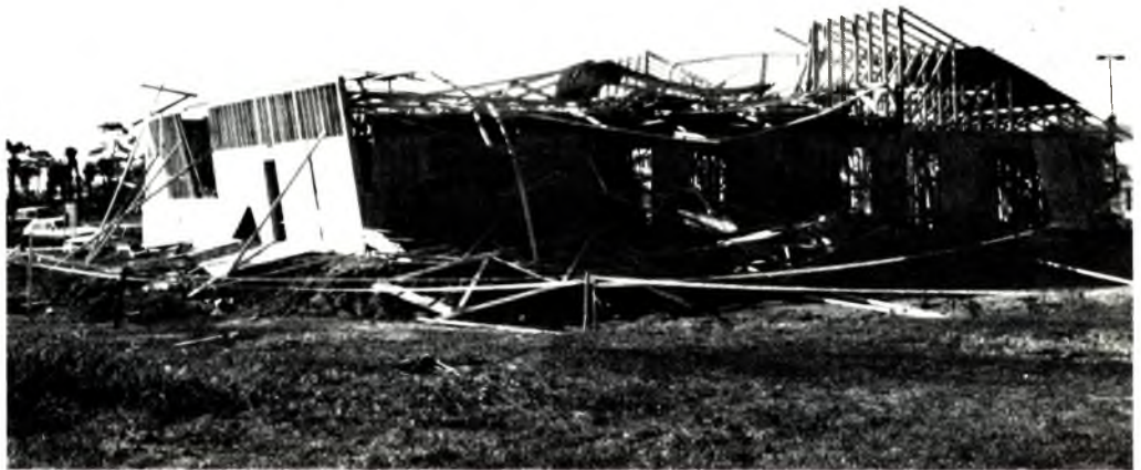
The Merritt Island, Fla., Church of the Nazarene, following damage caused by wind in mid-January
