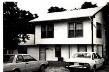
This house is one of 34 in Fort Worth that Liberation Community has renovated and sold to low-income families.
